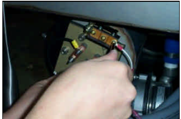
Securing jumpers to the thermostat.
